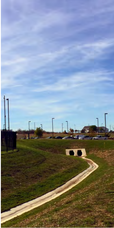
Smith Branch Flood Control - Williamson County
